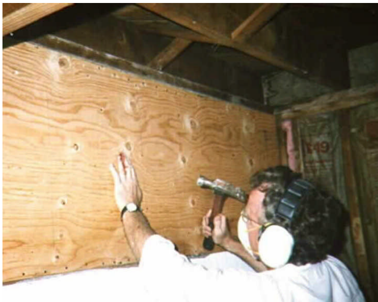
Figure 9 A structural panel installed to strengthen the pony wall to prevent the wall from collapsing, causing the home to fall off the foundation. (photo from Ben Emam, Amazon.com)
