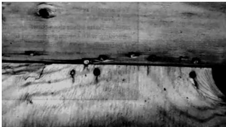
Figure 12 An example of overdriven nails and nails too close to the panel edge. Nails should be driven flush with the surface of the structural panel.
